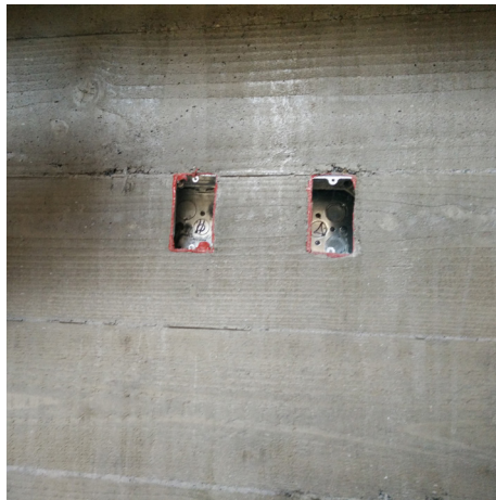
Above: one of the shear walls above the third floor slab. This wall is not exposed to the interior, so boardform was not used.
