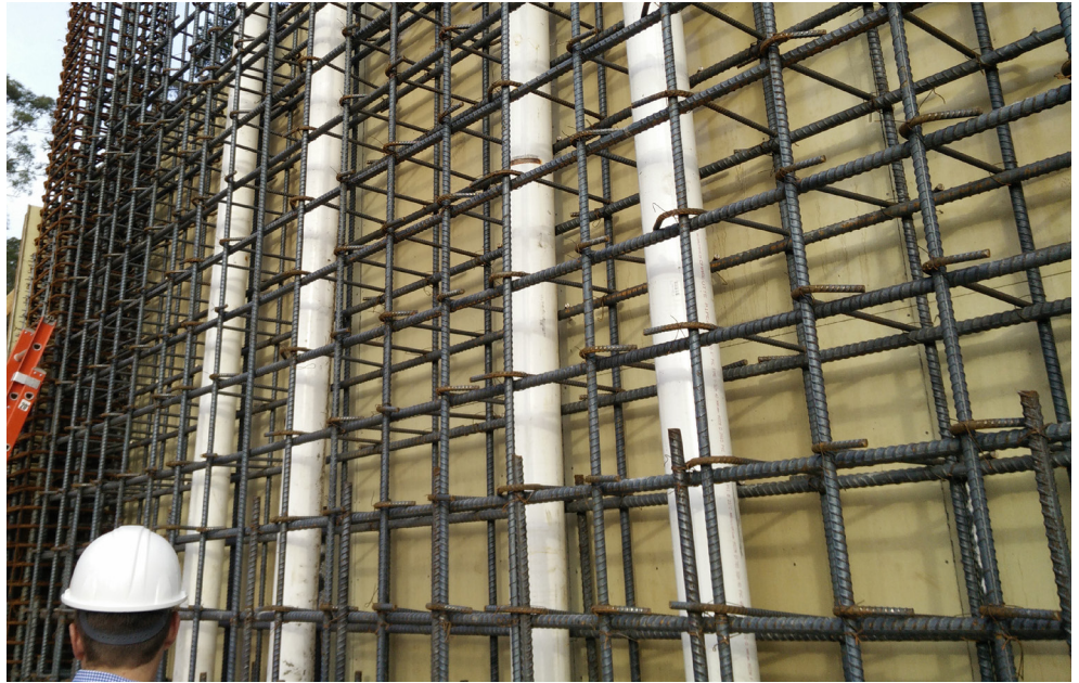
Above: one of the shear walls above the third floor slab. This wall is not exposed to the interior, so boardform was not used.
